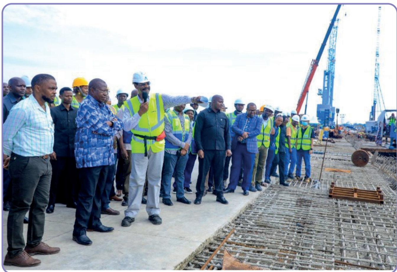
Vice President Dr. Philip Mpango (second-left) listens to explanation on Tanga Port improvement works by Niras Company's consultant, Eng. Abdallah Mwinyi, November 20, 2022 (Photo by Vice President's office (www.vpo.go.tz))
